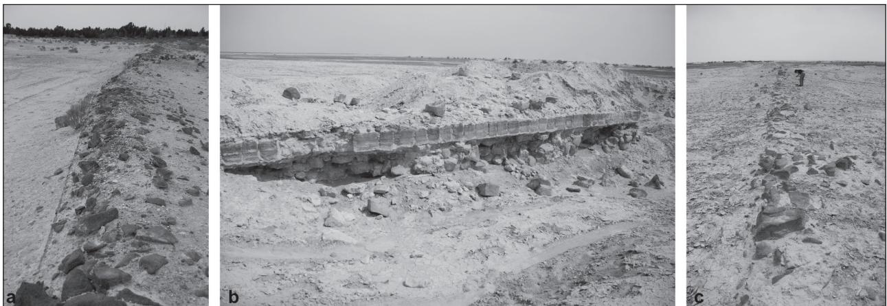
13. The long wall located south of the reservoir-enclosure and its different states of preservation: a) with the facing preserved; b) with the facing damaged causing collapse of internal fill; c) badly preserved (AASRP 2016).
