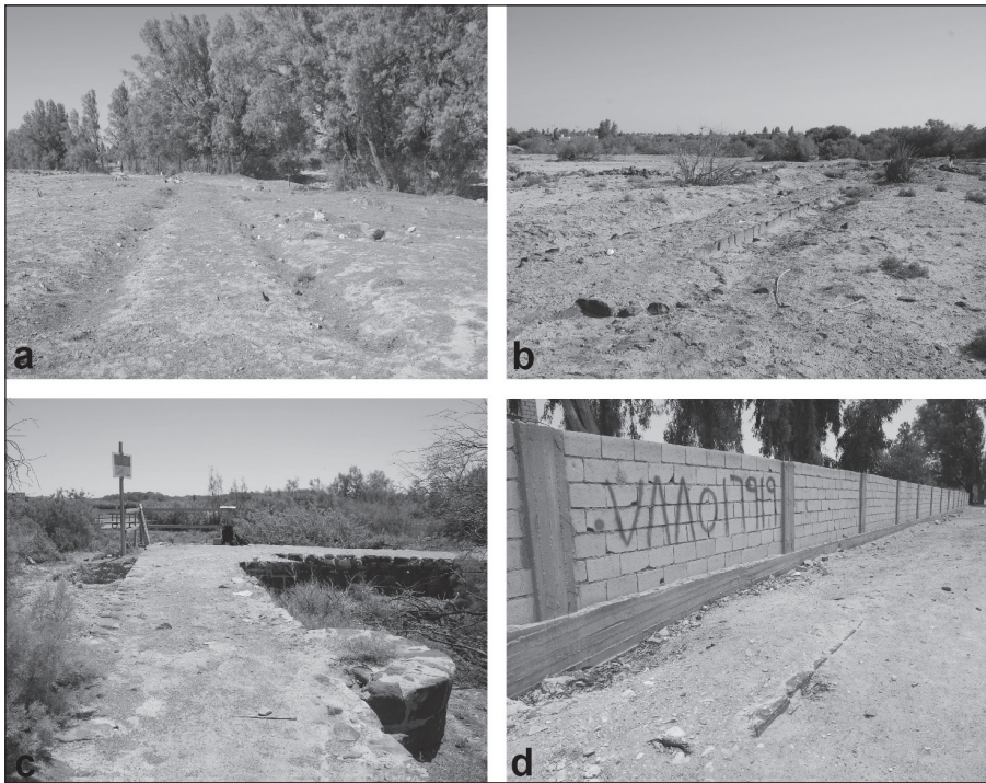
19. Views of different states of preservation of the architectural remains of the reservoir-enclosure: a) in section 1, the wall is located inside the Wetland Reserve, recognizable because of the topography of the terrain, but no longer visible; b) in section 2 (zone I), the wall is located inside the reserve but out of the tourist track and has not been restored; c) in section 11 (zone II), the wall is located inside the reserve, on the tourist track, and has undergone some modern restorations; d) in section 19 (zone III), the wall is located outside the reserve, on non-fenced properties (AASRP 2015).
