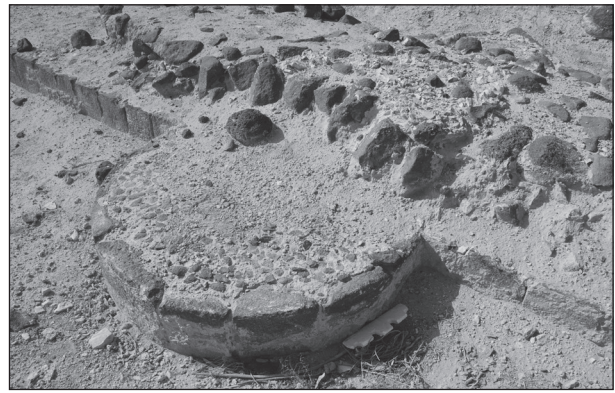
6. Example on the wall of the reservoir-enclosure showing the internal fill linked with the one of the buttresses (AASRP 2015).
