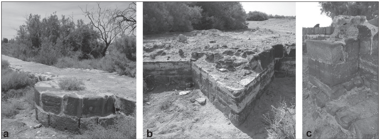
7. The three types of buttresses: a) semicircular; b) triangular; c) rectangular (AASRP 2014).
