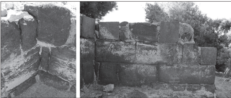
11. Two examples from Massif C showing the link between the wall and the buttresses: facing blocks penetrating into the main wall's masonry (AASRP 2015).
